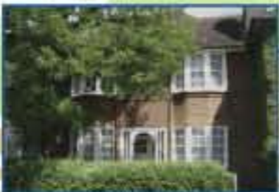
Tower Gardens Estate , council estate built 100 years ago as a 'garden suburb' - now a conservation area. Tower Gardens Residents Group: www.towergardens17.org.uk
